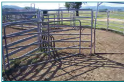
Bad corners in yards which have to be blocked off, caused in part by the gate hinging the wrong way (because the gate will only swing 90 degrees)
