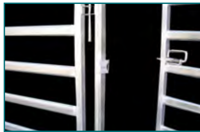
Bruise or cut points as stock pass. Under pressure this gate frame will bend and render the slam catch useless. Also gate can fly straight past the keeper.
