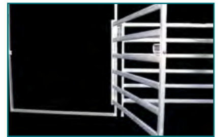
This is as far as the gate will open. This results in gates broken off their hinges due to the massive fulcrum effect if a beast hits or backs into a gate
