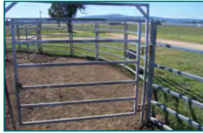
Gates hinged on outside of the yards result in poor stock flow and unnecessary walking for the operator
